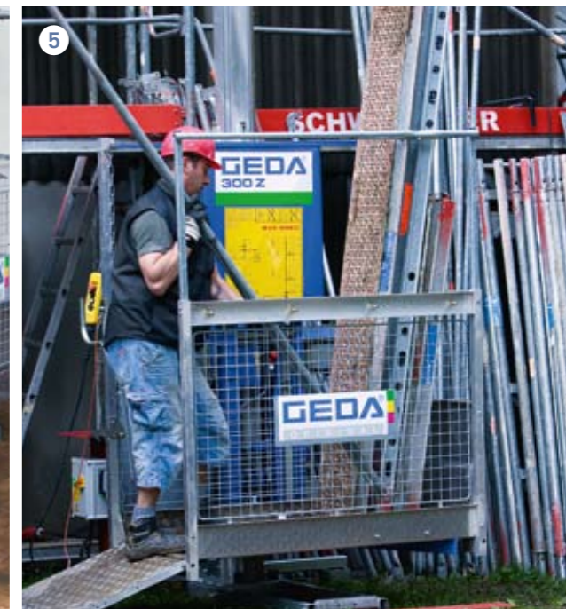
5 Scaffold frame enables safe transport.
